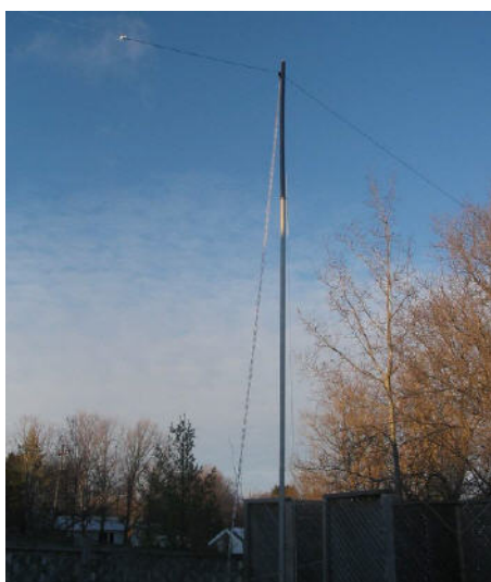
A good tidy G7FEK installation. This neat and tidy job is by Scott, VE3SCP. This is a 24ft vertical section with 8 and 38ft horizontal extensions.
