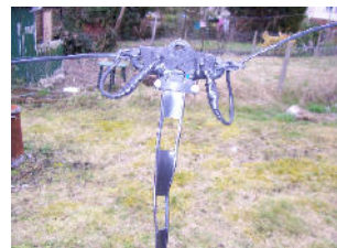
At the top of the feeder, after weather-proofing - not pretty but waterproof!!
